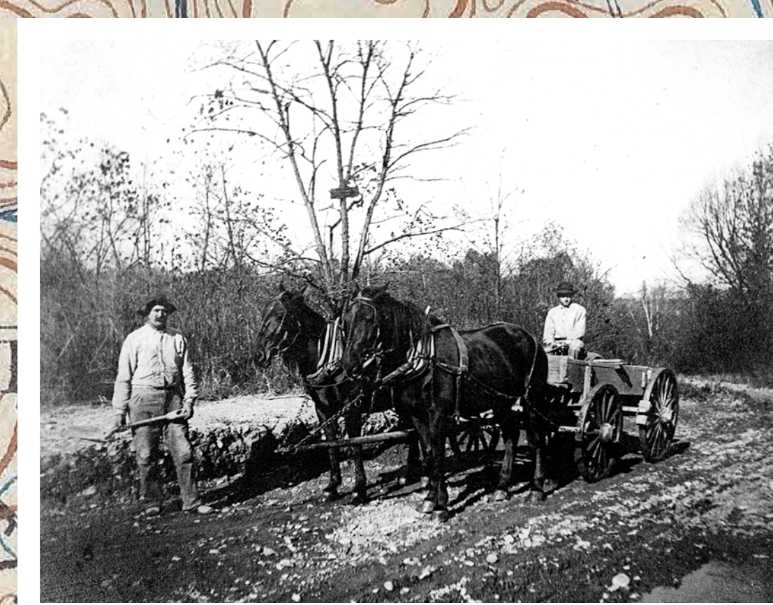
Lawrence Leuser and William Kuntz haul gravel from Clough Creek near Clough Pike and today's Berkshire Road for road repairs around 1915.
