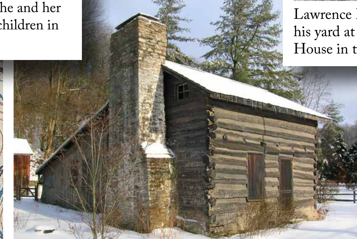
The Miller-Leuser Log House still on its original site. It is owned by the Anderson Township Historical Society. Photo from 2015. By C. Wallace.
